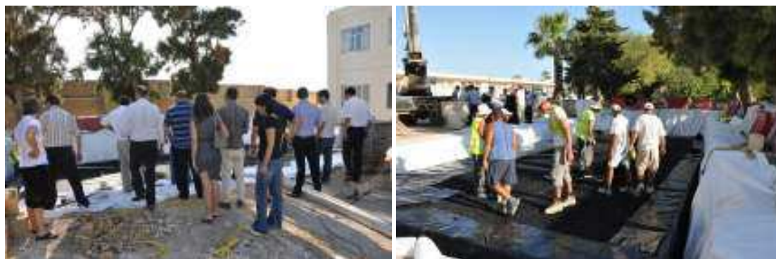
Site visit & on-the-job training for local technicians and professionals in the construction industry.
